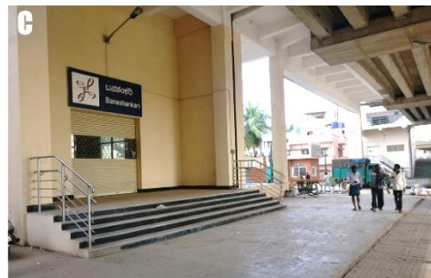
Figure 24: Access point C
