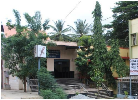
Figure 9: Access point C
