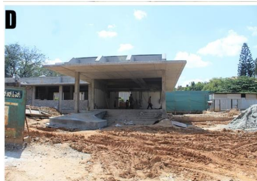
Figure 62: Access point D
