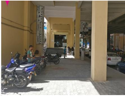
Figure 40: Access point B
