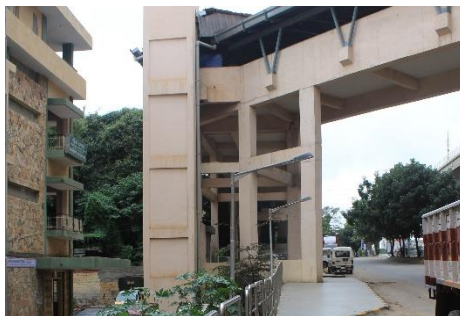
Figure 7: Access point B
