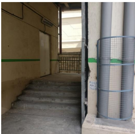
Figure 34: Access point C
