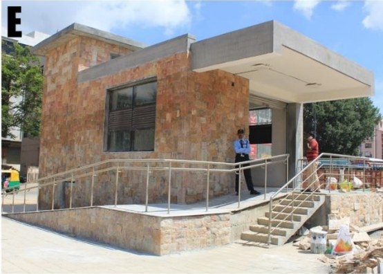
Figure 63: Access point E
