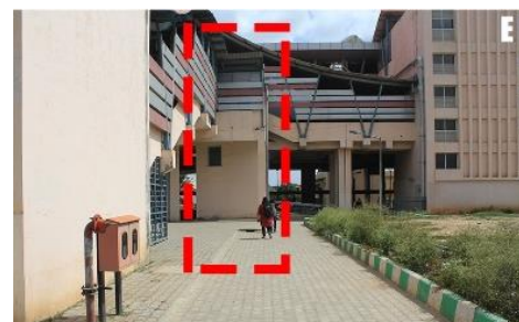
Figure 13: Access point E
