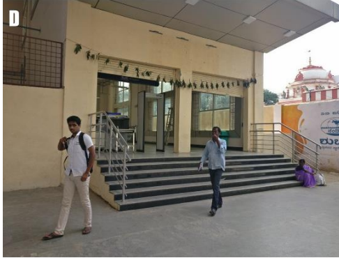
Figure 25: Access point D
