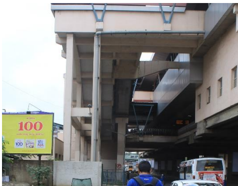
Figure 11: Access point D
