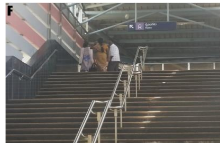
Figure 15: Staircase at access point F
