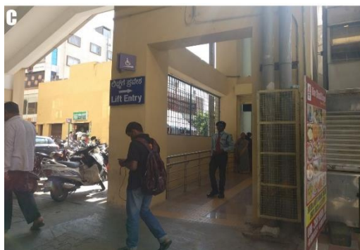
Figure 42: Access point C
